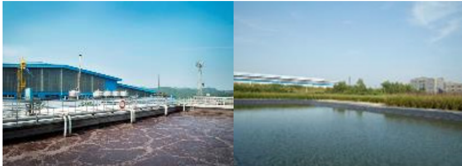
WWTP and Wetlands of China facility
