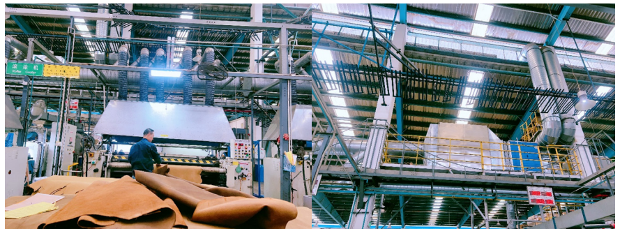
New activated carbon absorption device for VOC treatment at finishing of China facility (HTL), including exhaust gas collection cover for roller coating.
