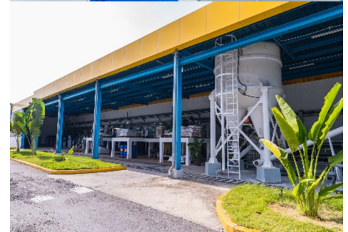
WWTP of Vietnam facility
